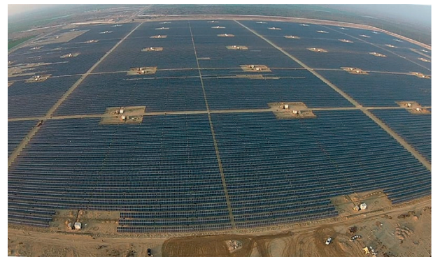
FIGURE 2: An aerial view of Quaid-e-Azam Solar Power Park.
