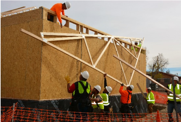
UNM-G Construction Technology Students Working on Habitat for Humanity House
